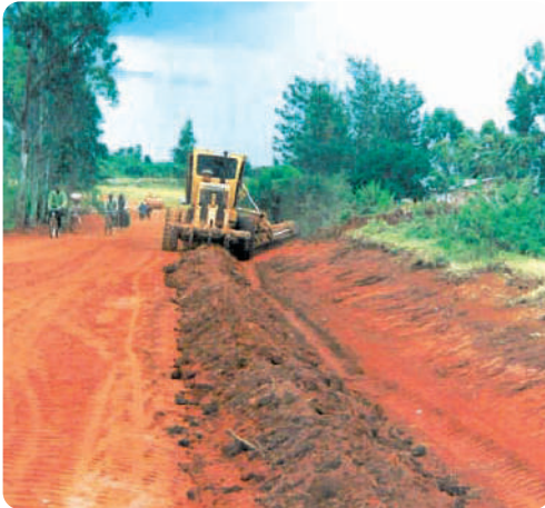
Fig 4.5: A tractor destroying land to give space for road construction
